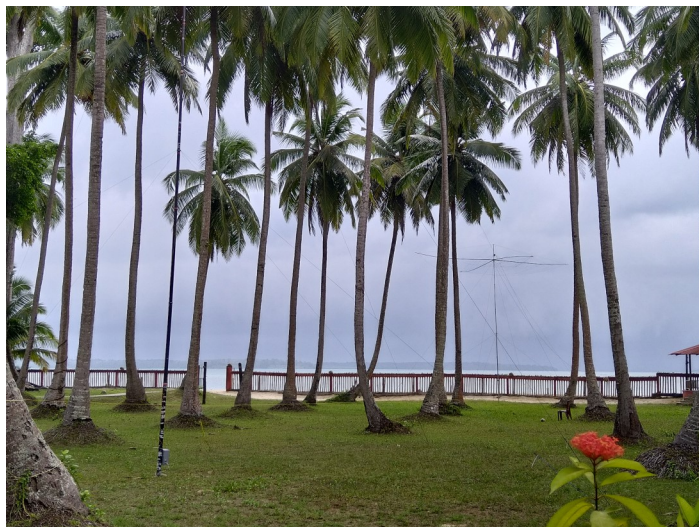
Yard with antennas
