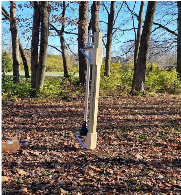
Figure 5 4x4, rotor, and thrust bearing on "tower" portion. Looks crooked but it isn't!
