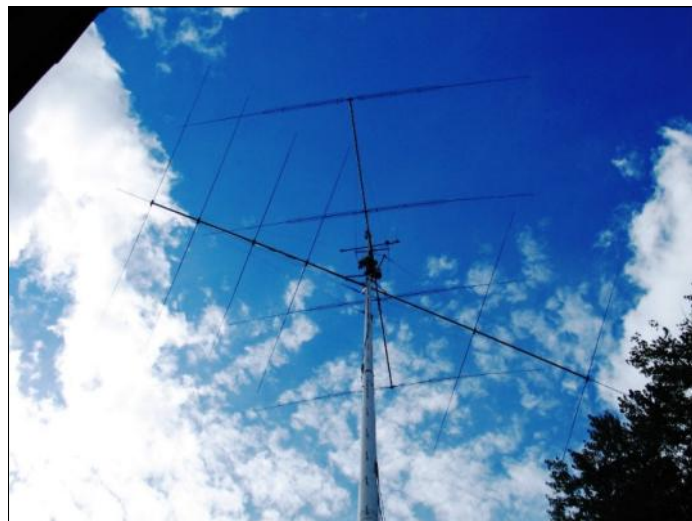
Lowering the KLM 6-element 20 meter Yagi.
