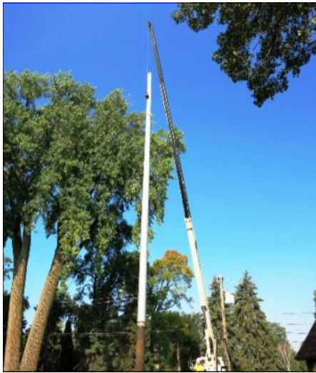
Lifting tower out of base tube.
