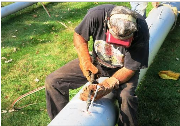
Cutting tower into 30-foot sections.
