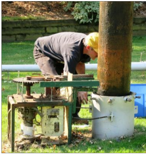
Removing bolts from base tube.
