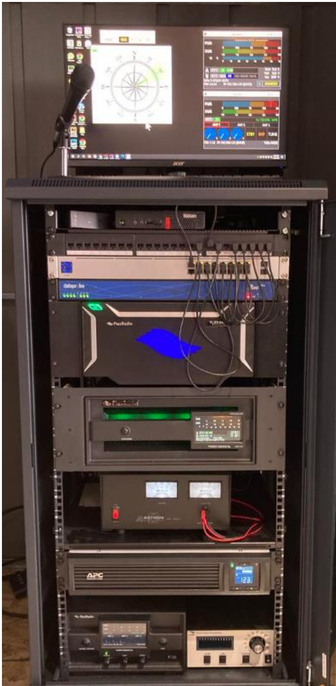
In the Rack From top to Bottom: TempStick, Lenovo PC, Network, PDU, Flex 6400, Flex PGXL, Astron Power Supply, APC UPS, Flex TGXL, Green Heron RT-21
