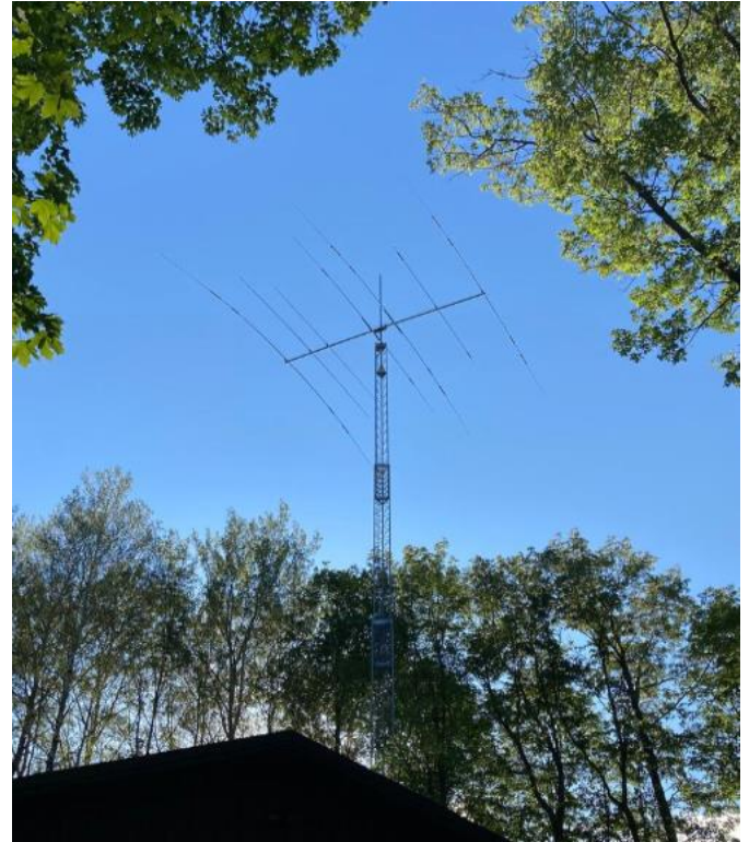
Mosley PRO-67-C-3 at 75 feet/25m [3 elements on 40/20/17/15/12 meters; 4 elements on 10 meters]
