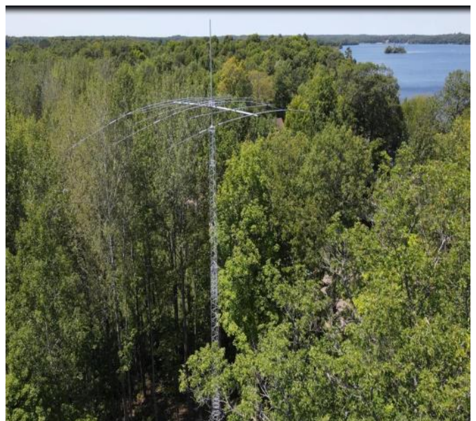
Mosley PRO-67-C-3 at 75 feet/25m [3 elements on 40/20/17/15/12 meters; 4 elements on 10 meters]
