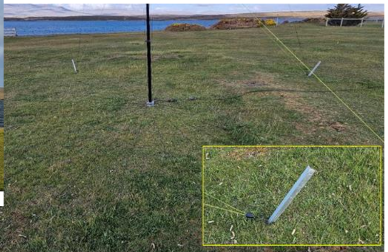
Figure 6 - 32 radials, 3.5 meters long and extra-large guy anchors.
